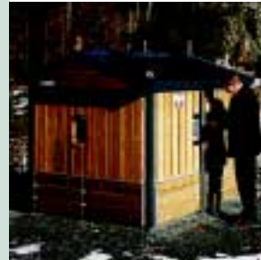
Compact secondary substation
